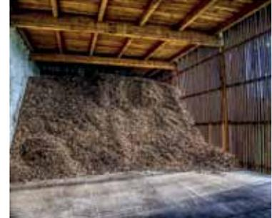
Wood chip bearing of a local heating network.
