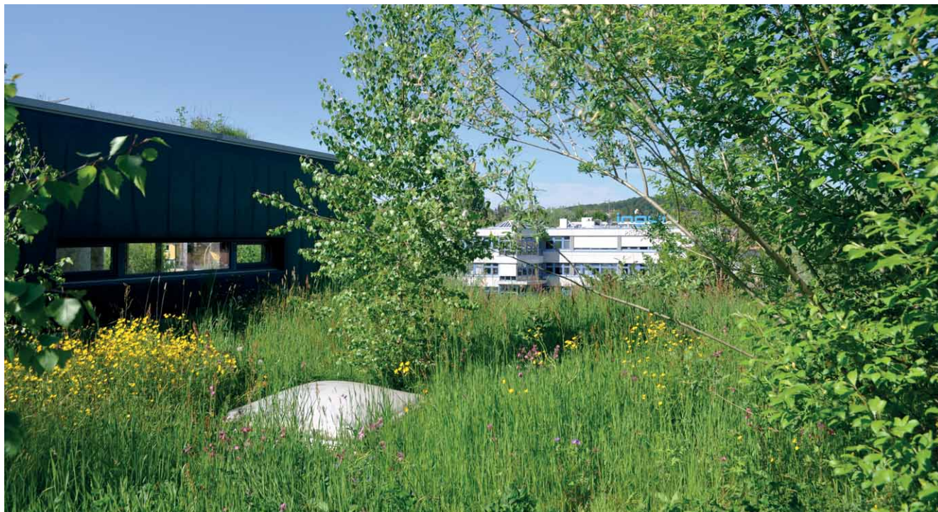
Green roofs can save energy for air-conditioning and offer habitats.
